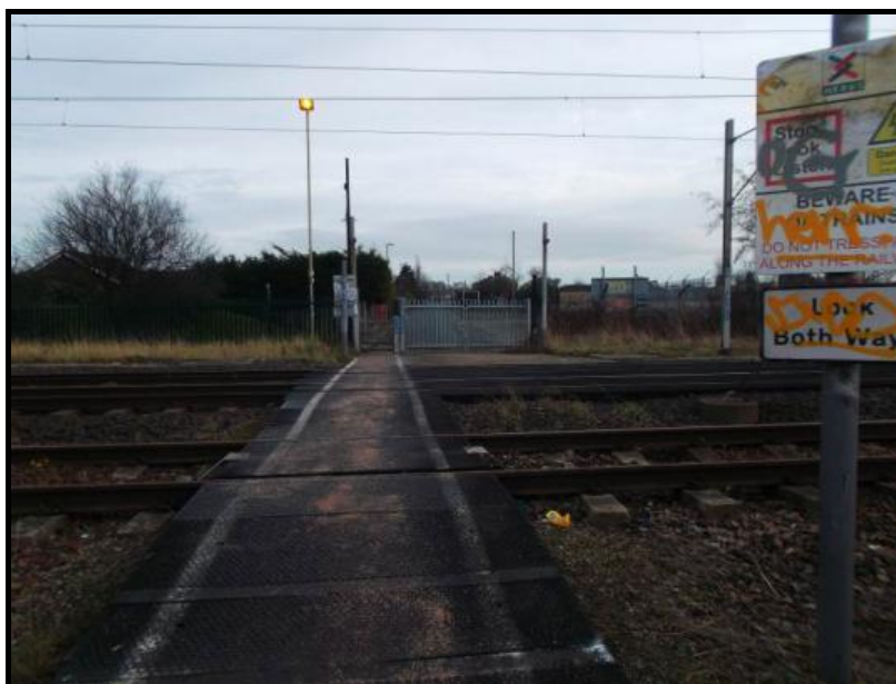
Photograph illustrating length of crossing and signage obscured by graffiti
